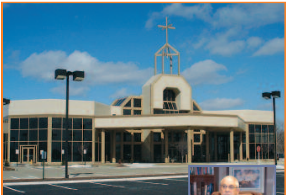
First Assembly of God Church in the former Behlmann Auto Dealership building
